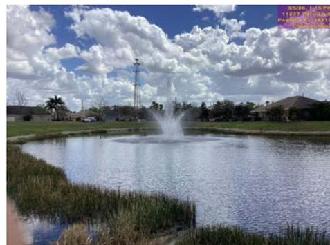
Fountain has been cleaned / pressure washed and flushed, intake screen cleared, all components inside control box as well as clocks/timers checked.
